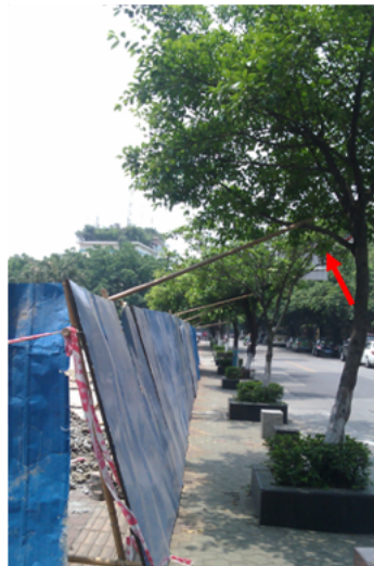
Figure 3: Using tree as anchor may damage its bark.
