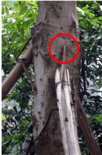
Figure 4: No nails shall be driven into the tree as it promotes infiltration of pests/diseases
