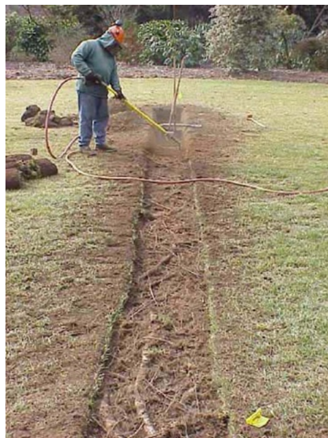
Figure 10: Root exploratory works using an air spade. Air spading avoids damage of structural and even feeder roots of the tree.
